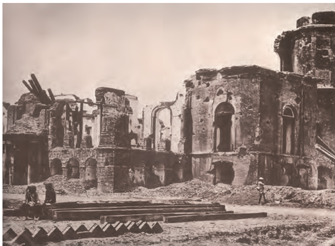
Fig. 17 – Ruins of the Residency in Lucknow
